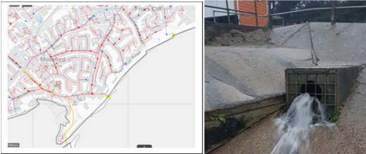
Surface Water Outfall: Local Map and at Steamer Point
